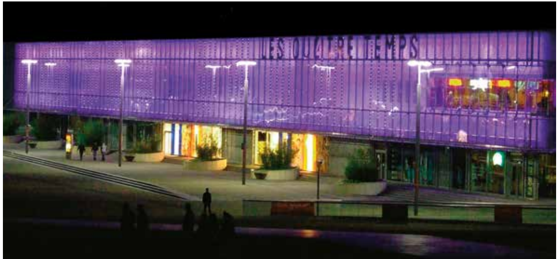
Illumination of the facade of Les Quatre Temps shopping center (Paris La Defense), lighting design by Voyons Voir, performed by VD by using 500 MODULED 150 RGB projectors.
